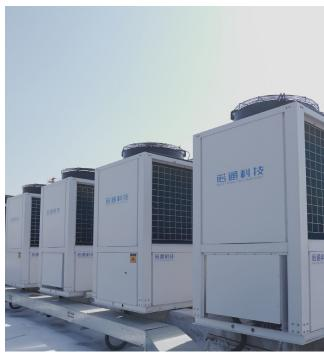
At low-temperature (room temperature, outlet water temperature below 60°C), the project specially designed a heat and cool balanced air-source heat pump heating and cooling unit (170 kW) based on Copeland's ZW286 compressor to heat and cool the factory's operation center and aerial garden-style building.
